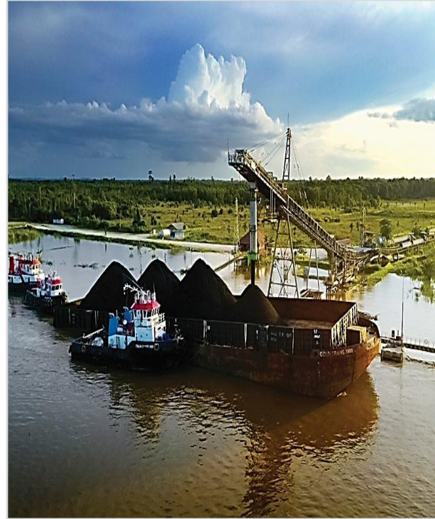
Improvement in Bunyut Port facilities and coal logistic capacity expansion (port stock yard expansion) at Melak
